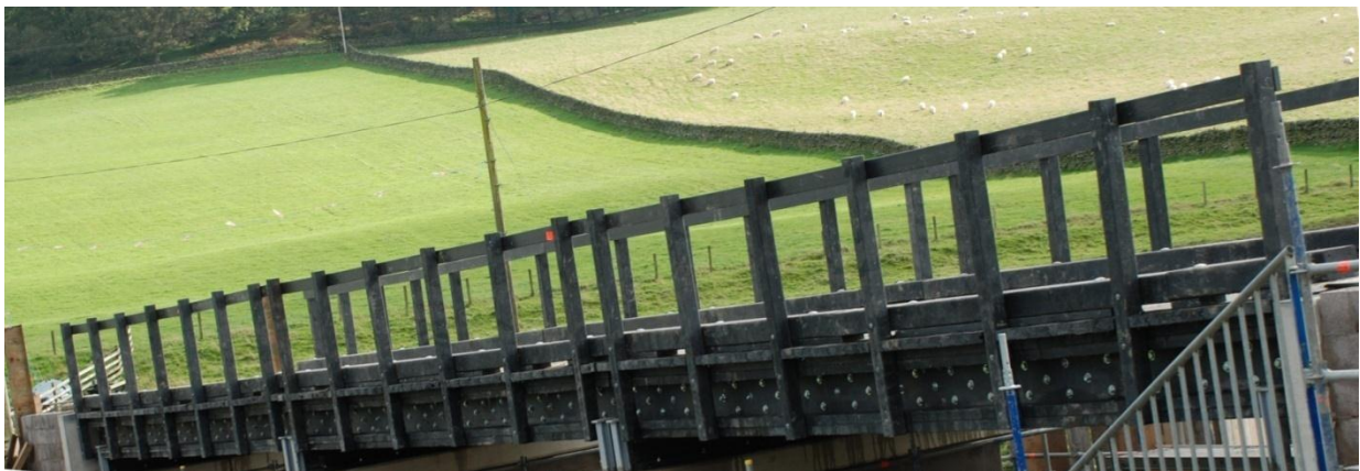
The completed 30 metre bridge
