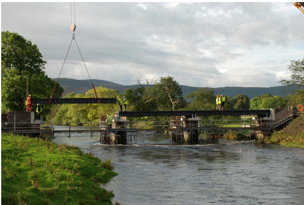
Final Span being craned into place
