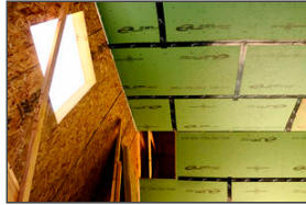
Gordon Chibroski/Staff Photographer Waterproof, insulation-grade heavy wallboard is meant to keep heat from escaping through the ceiling and attic.
