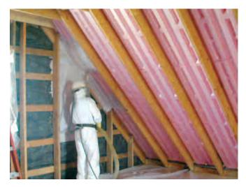
Corbond spray-on foam insulation has an R-value of about 7.3 per inch.
