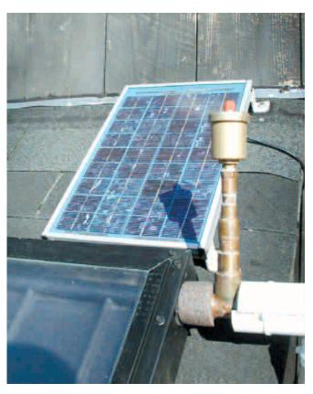
The air vent shaded the PV panels in the early morning, causing a delay in pump operation—Oops!
