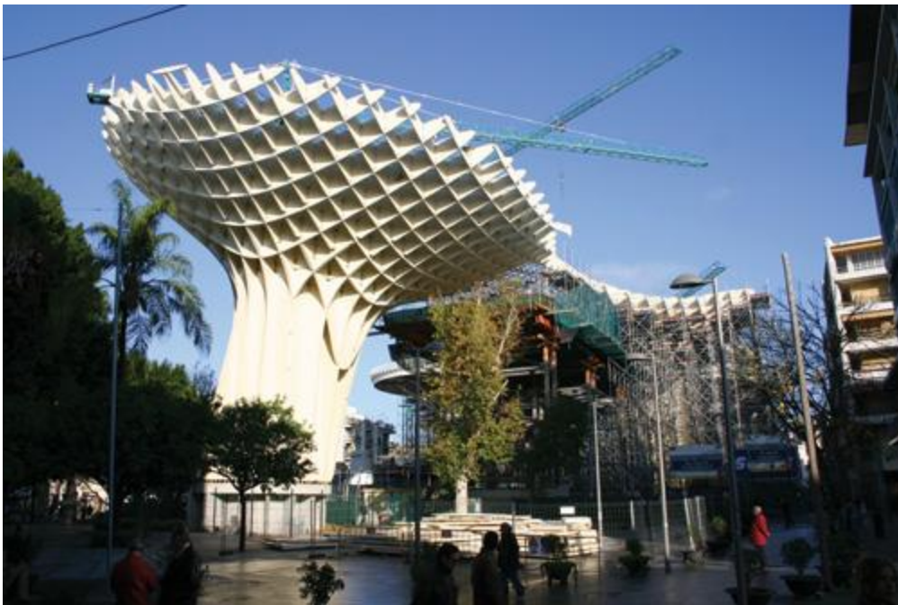
Phase 5: Scaffolding down
