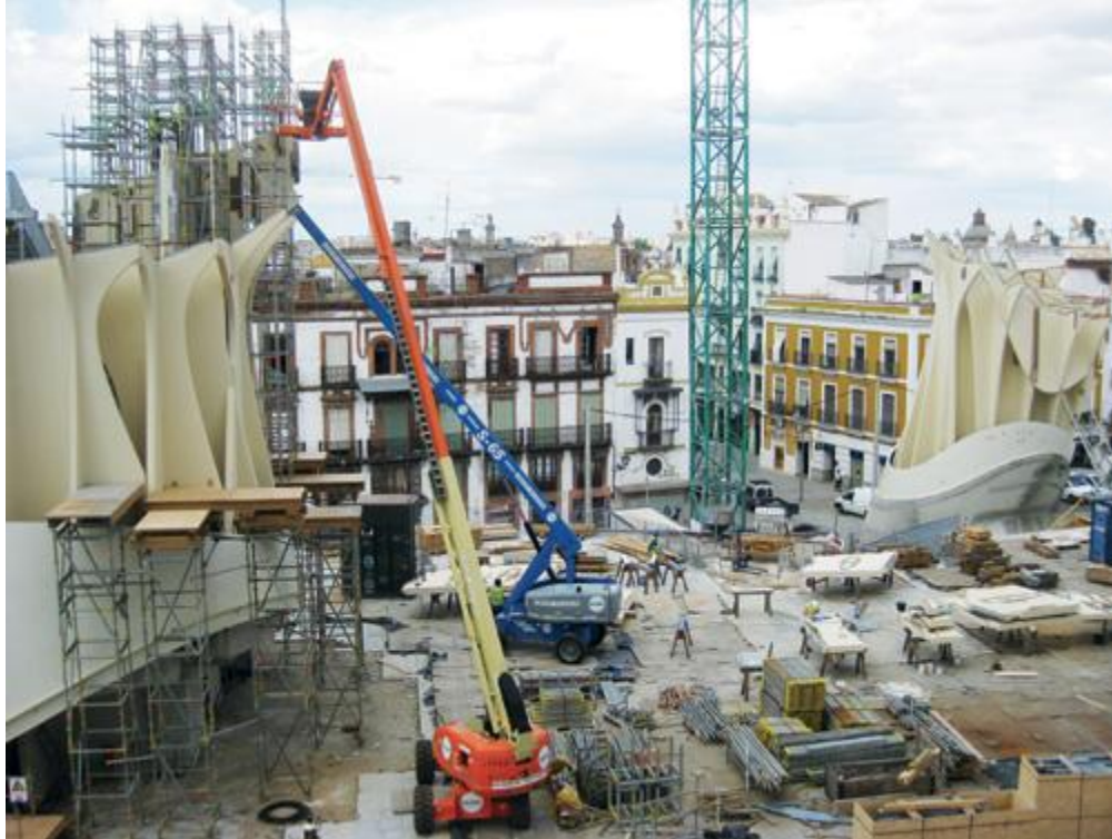
Phase 3: Main structure
