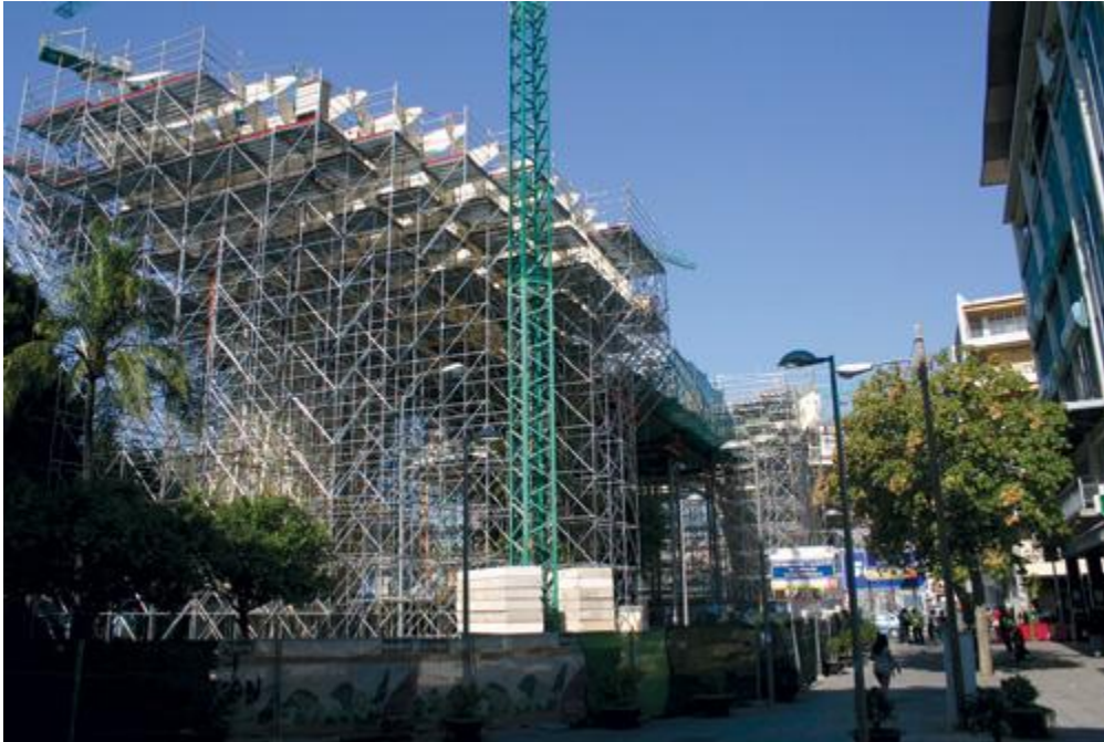
Phase 4: Scaffolding up
