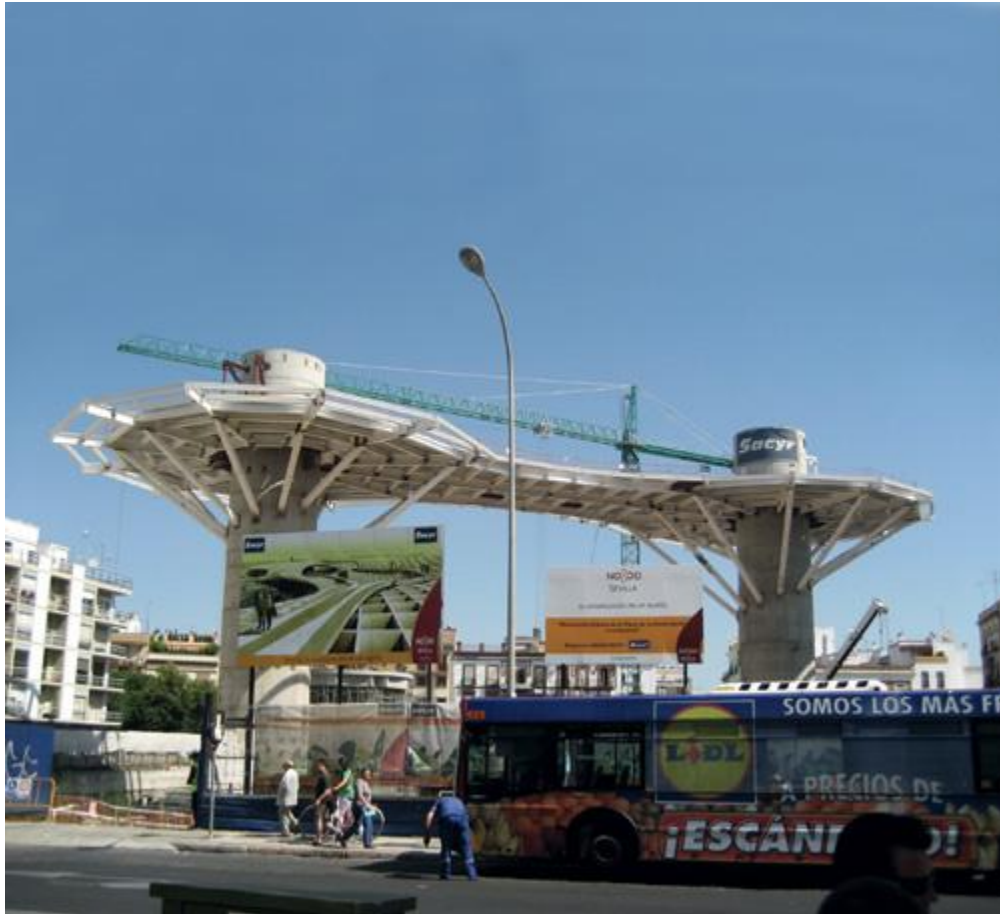
Phase 1: Concrete structure
