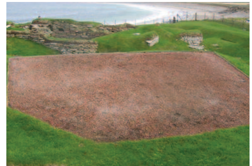
Ground preparation prior to installation
