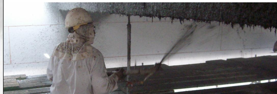
A structural beam is coated with glass fiber reinforced concrete using spraying equipment for a commercial warehouse in Scottsdale Arizona.
