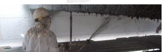
A structural beam is coated with glass fiber reinforced concrete using spraying equipment for a commercial warehouse in Scottsdale Arizona.
