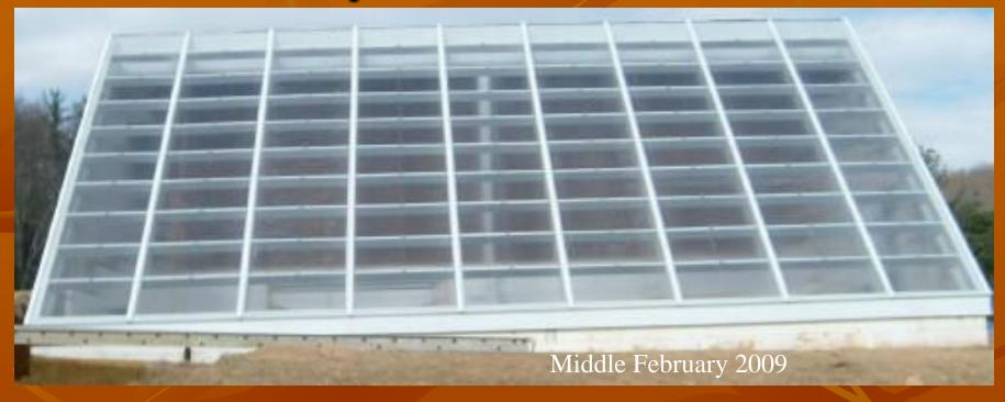
20' long x10-mm thick double-walled polycarbonate with ribs separated by 1 cm.
