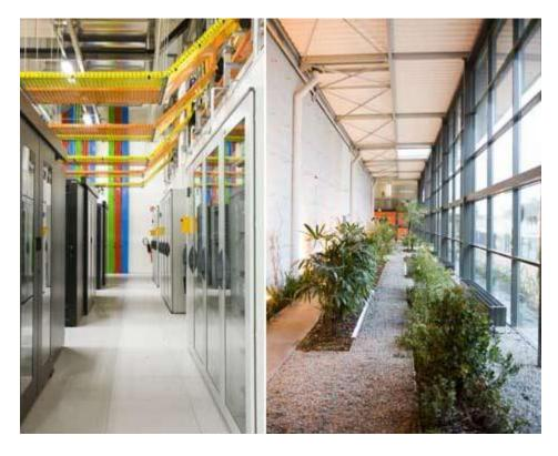
Waste heat from servers at the new Telecity Paris data center (left) is being used to heat an on-site arboretum (right).
