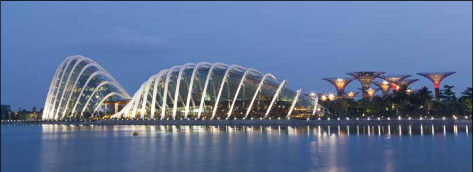
The Cloud Dome and Flower Dome. Paul Baker of Wilkinson Eyre Architects says: "The complementary yet distinct curved forms of the biomes are generated from the geometry of a hyperbolic curve, and so contain a large volume within a relatively small surface area. Not only does this geometry enable the structure to be optimised (allowing a lightweight, column-free interior), it works well environmentally, creating a stack-effect with warm air drawn up to stratify according to temperature within the space. The gentle forward tilt of the Flower Dome towards Marina Bay also shades the north façade so it never receives the full impact of the sun." © Craig Shepherd
