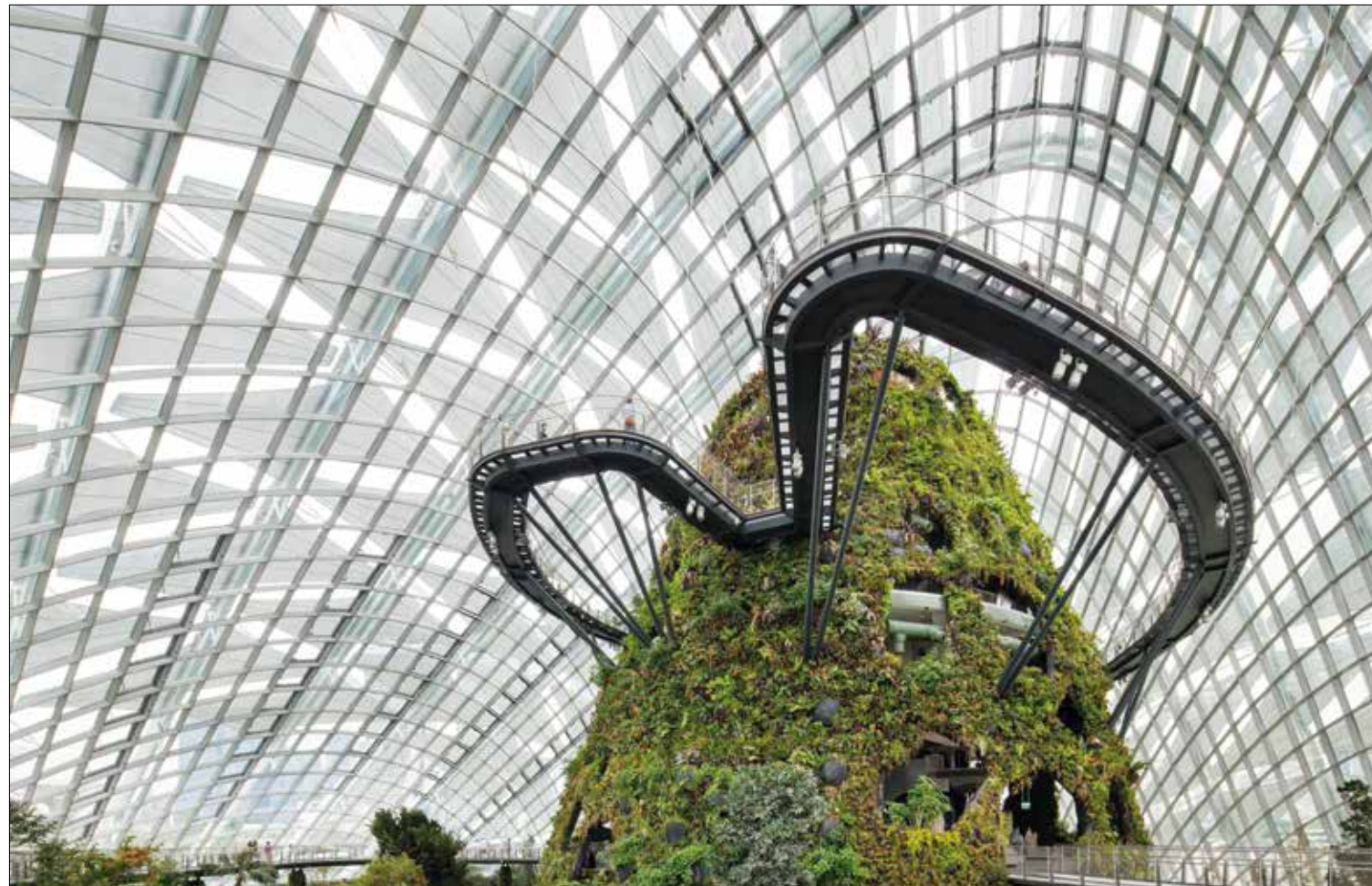
In the Cloud Forest, looking up at the artificial mountain with its vertiginous aerial walkways. Above the slender grid shell roof, the triangular shades have been deployed to protect the plants from tropical sun © Craig Shepherd
