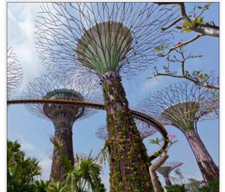
As well as holding ferns, vines, orchids and also a large collection of bromeliads, the Supertrees are fitted with environmental technologies that mimic the ecological function of trees. There are photovoltaic cells that capture solar energy which can be used for functions such as lighting and the collection of rainwater, used for irrigation and fountain displays. They also serve as air intake and exhaust functions, part of the conservatories' cooling systems with an elevated walkway between two of the larger Supertrees © Craig Shepherd
