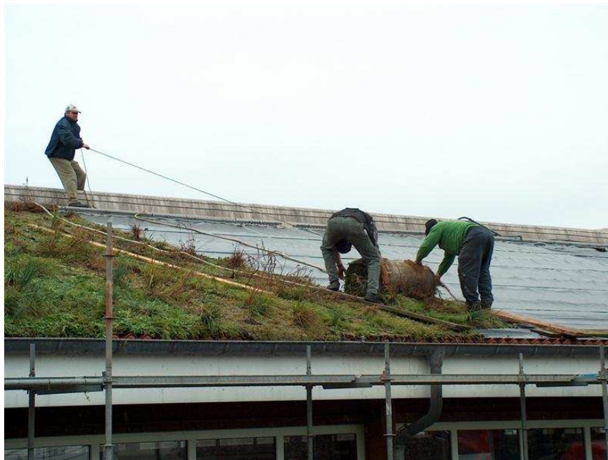
Installation of the plant mats
