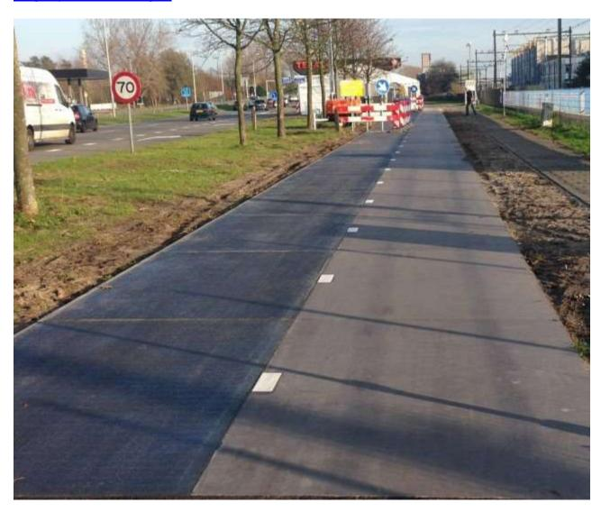
At present, only 70 meters of a planned 100 meters has been completed and only one side. This stretch of path is bathed in consistent sunlight for most of the day, making it a good test case for the project. In the image above, the solar road is on the left, the traditional concrete is on the right.
