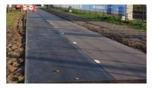
Earlier this week, the first solar roadway opened in Amsterdam — a 70-meter stretch of cycle path between two suburbs of the city that generates solar power from rugged, textured glass-covered photovoltaic cells. My significant other, Jessica Hall, happens to be spending a semester in Amsterdam and was willing to trek out to the Krommenie-Wormerveer cross-connection to see this solar roadway in action.
