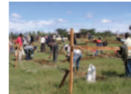
TOP LEFT Staking out the site for the rainwater court. Photo: Greg Elsner/Architecture for Humanity
