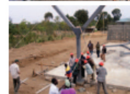
FIFTH FROM TOP LEFT Wire cage framing for the water cistern with a capacity of 15 000 gallons. Photo: Greg Elsner/Architecture for Humanity
