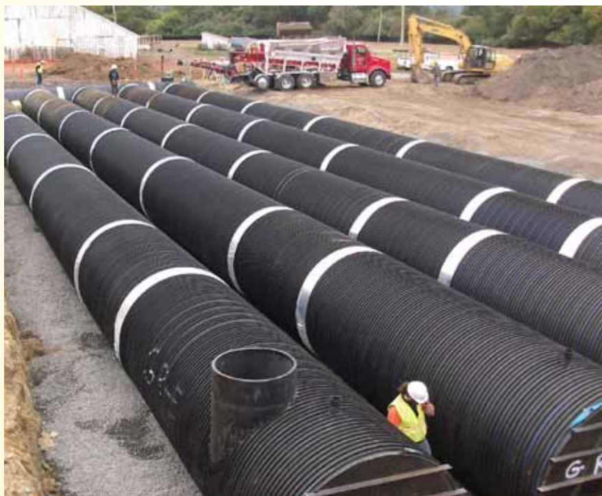
Figure 2: An underground SRPE cistern is installed in California, 50 percent backfilled with stone.
