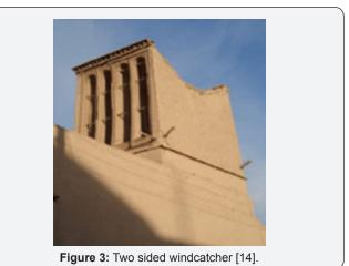
In regions with strong predominate wind, two-sided wind catcher is generally utilized which have two vents and two distinct underneath halves. Figure3 shows the bidirectional wind catcher is separated into two channels in order to supplying (suction) and extraction of air flow.
