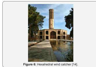
These types of windcatchers have been usually seen with regular multifaceted plans and they were designed in the shape of hexagon or octagon. Generally, they are higher than other windcatchers, especially eight-sided windcatcher; therefore, they will have more stability against wind pressure as well as tower form causes passing air flow with lower pressure.
