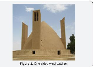
In other words, if there is an unfavorablewind directions, one-sided windcatcher will not well function. Hence, inlet openings of windcatcher should be at as much as high level to enjoy stack effect (buoyancy effect) like a solar chimney function for that special condition. Figure 2 depicts the structure of onesided windcatcher, the wind goes in from the single opening and passes via the living space and leaves the exhaust vents, doors, and windows.
