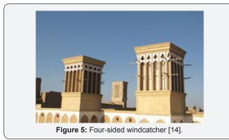
Based on previous studies, an abundance of four-sided windcatcher is more than other types of this system in the Middle East. In areas where there is no specific direction for wind, foursided windcatcher can be seen; therefore, its design is mainly dependent upon capturing the wind from all directions. Foursided windcatchers with decorations belong to a famous family's house in the city of Yazd, Iran as shown in Figure 5 [8].
