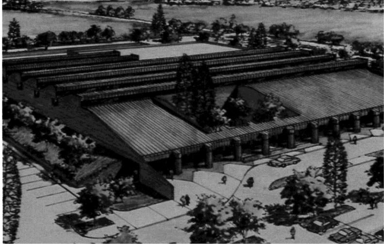
**Figure 1-24: Monitor Apertures. Commissary, Vandenberg AFB, California**
