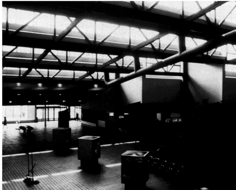
Figure 1-5: Direct Gain. Walker Field Terminal, Grand Junction, Colorado
