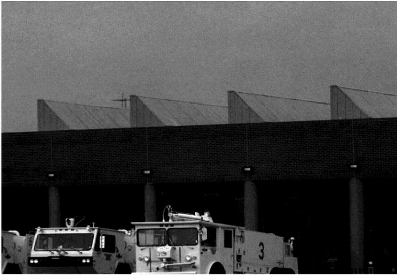
**Figure 1-22: Sawtooth Apertures. Fire Station, McEntire A.N.G. Base, South Carolina**
