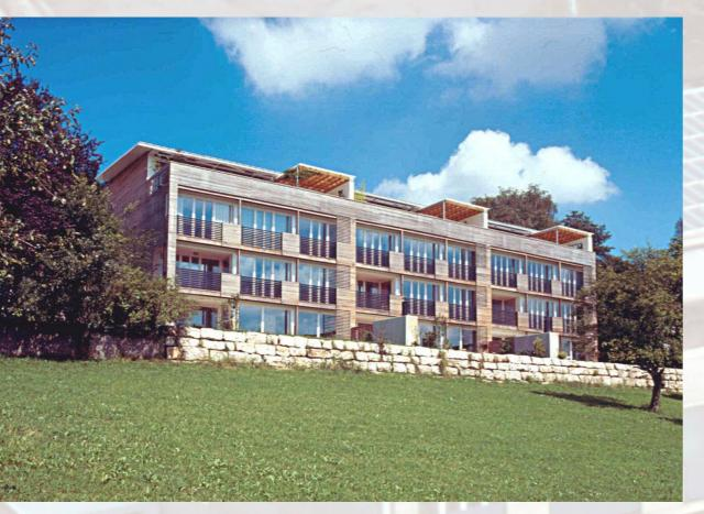
Sunny Woods was erected using a brand-new timber technology. As one of first 4 storey apartment buildings in Switzerland it was constructed with timber only. The timber elements were manufactured at a carpentry to exact dimensions. It was extremely quick and easy to assemly them on site. The external walls of approximately 40cm thickness consist of a load bearing blockboard of only 3.5cm, leaving plenty of space for thermal insulation.
