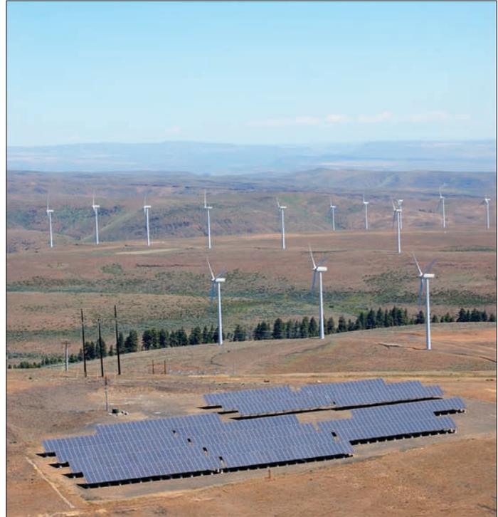
At 500 kW, the Wild Horse solar array is the Northwest's largest demonstration project of photovoltaic technology, which turns sunlight into electricity.
