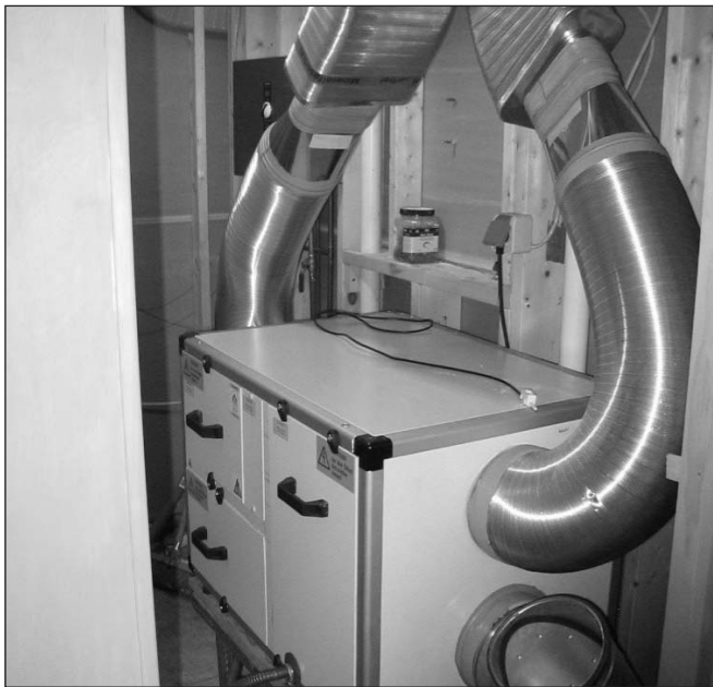
Figure 4. The Westaflex WAC 250 is a heat-recovery ventilator that can control dampers that select between two possible air intake ducts, depending on the outdoor temperature. It also includes a 1,000-watt electric resistance element to heat the house.
