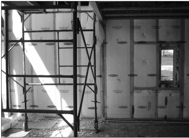
Figure 3. The 12-inch-thick walls were insulated with Optima blown-in-place fiberglass insulation.
