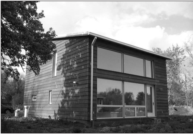
Figure 1. Architect Katrin Klingenberg's superinsulated house in Urbana, Illinois conforms to standards established by the Passivhaus Institut of Darmstadt, Germany. The house's simple, box-like shape minimizes its surface-to-volume ratio. On the west side of the house, the fresh air intake duct and exhaust duct can be seen where they emerge from underground.
