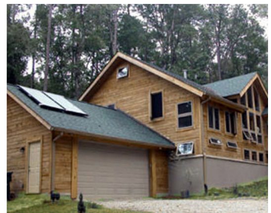
View showing solar hot water panels
