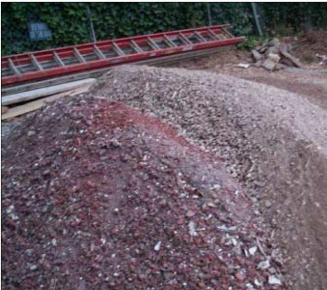
MR113 Site-Processed Materials (Brick, Fill) for Patio Block Base
