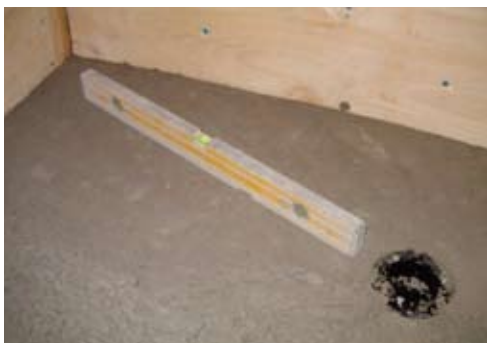
Durable shower pan, under construction
