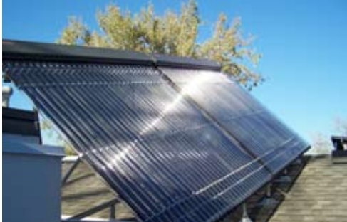
Evacuated tube solar water array
