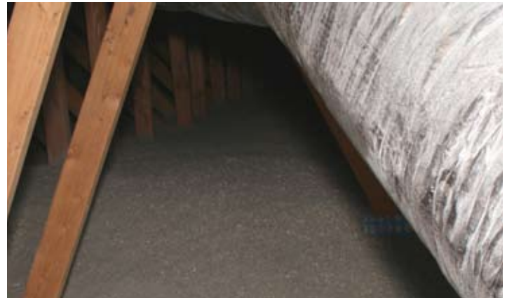
After: attic reinsulated with cellulose
