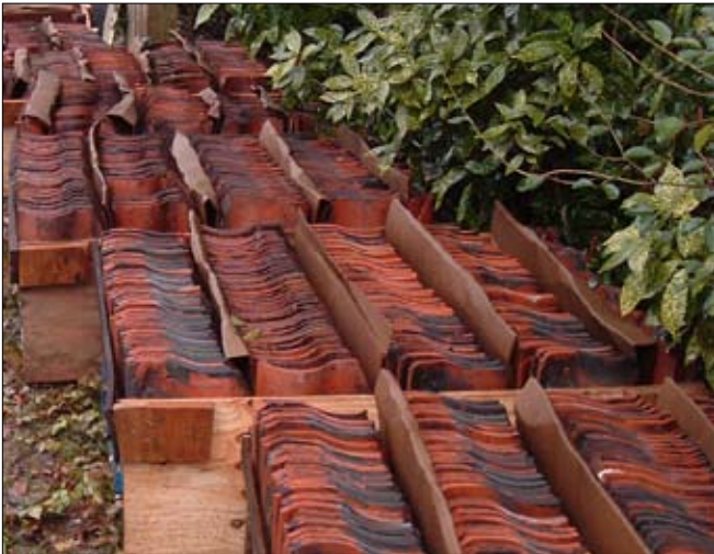
MR108 Salvaged Roofing Tiles Ready for Reinstallation
