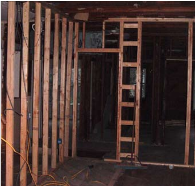
MR116 Advanced Framing on Interior Partitions
