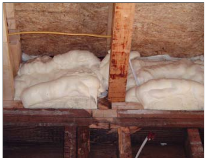
EA55 Spray-Foam Insulation at Rim Joists
