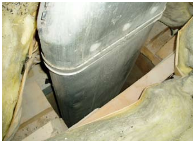
EA54 Thermal Bypass: Duct Chase
