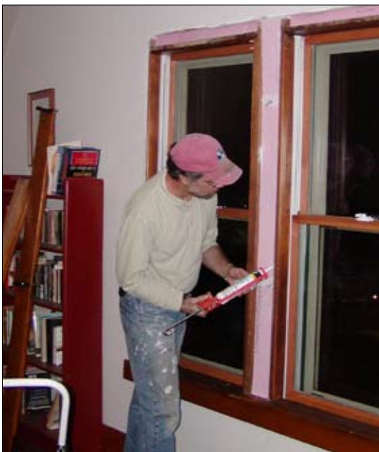
EA58 Interior Trim Removed to Insulate and Air Seal Sash Pockets after Sash Replacement
