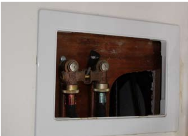
MR124 Single-Throw Clothes Washer Shut-Off
