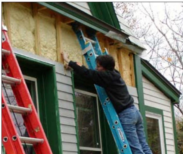
EA45 Exterior Wall Air Sealed and Insulated with Spray Foam; Reclad (Note Exterior Jamb Extensions Furring)
