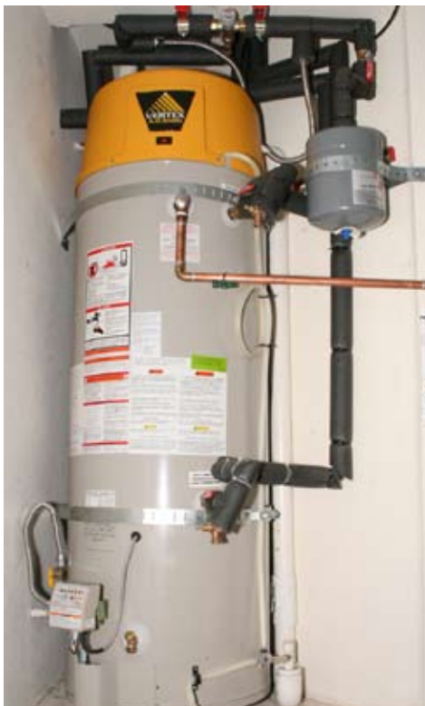
After: power-vented high-efficiency water heater
