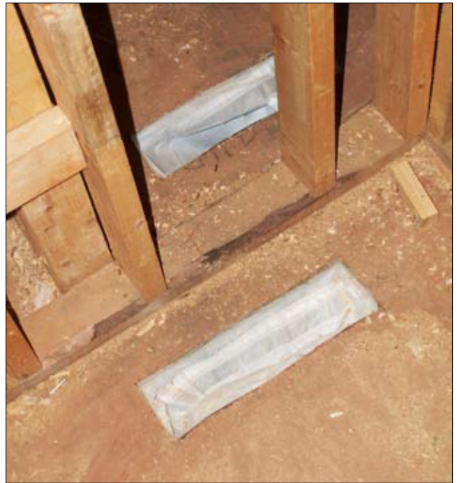
EA71 Duct Protection during Renovation
