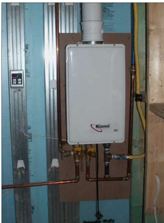
EA79 One Approach to Efficient Hot Water: Gas Tankless Heater
