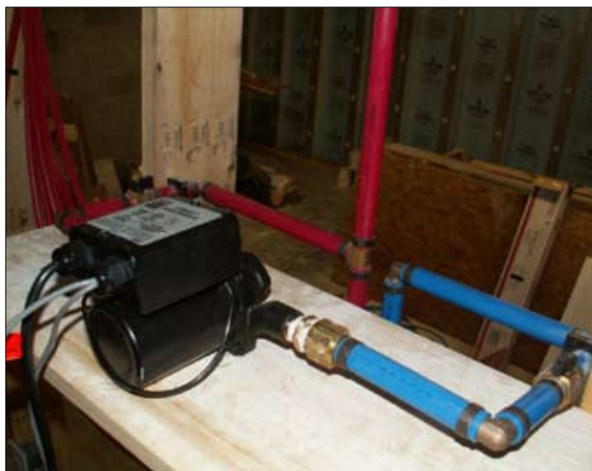
EA78 On-Demand Recirculation Pump for Hot Water
