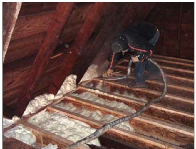
EA54 Spray Foam to Insulate and Air Seal
