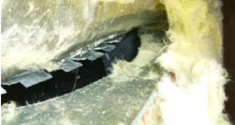
Before: duct leakage
