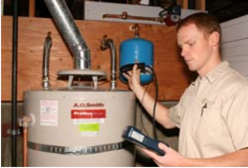
Home performance audit: testing water heater draft
