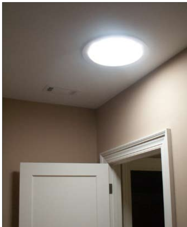
EA83 Solar Tube for Daylighting
