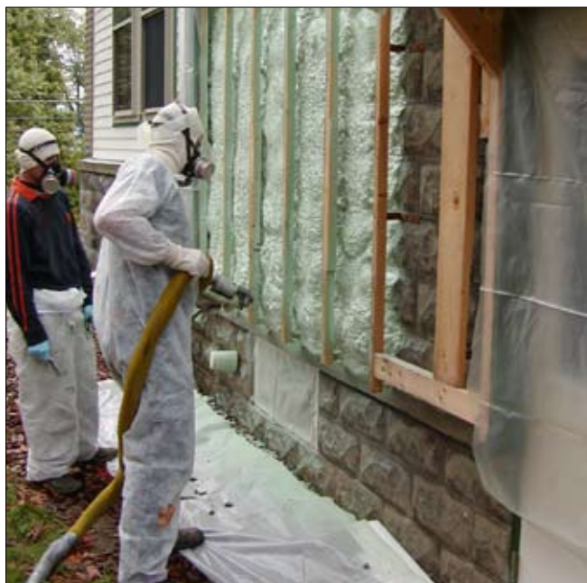
EA45 Exterior Wall Spray-Foam Insulation
