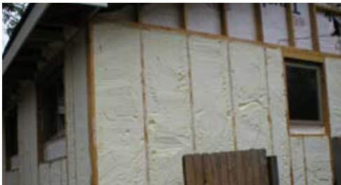
Spray foamed exterior curtain wall
