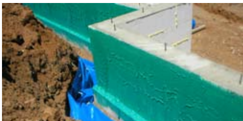
Water-managed, ICF crawlspace foundation
