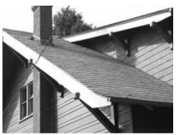
Recycled tire roofing on completed 1909 House
