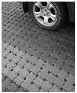
Pavers with open corners provide more formal appearance and rainwater drainage
