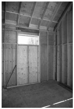
Efficient framing reduces non-structural wood
