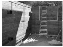
Form boards to be reused for floor structure
