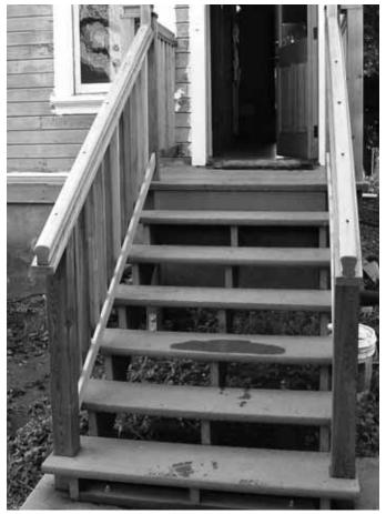
Stair treads made from recycled polyethylene and wood fiber
