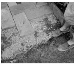
Rubble reused as base for permeable paving
