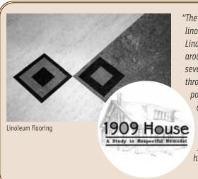
"The flooring is environmentally friendly sheet linoleum provided and installed by Lansing Linoleum. This long-wearing material has been around for the last 90+ years and has made several reappearances as kitchen flooring throughout the last century. Today it is very popular again mainly for its biodegradable content, durability and the range of beautiful colors it comes in. And for any you out there that HATE cleaning floors, the medium to dark colors seem to hide the dirt longer..."
