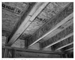
I-joists replace solid lumber joists
