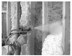
Spray-in Icynene provides complete cavity fill and is non-toxic
