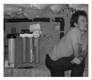
Particle and UV filters purify rainwater
