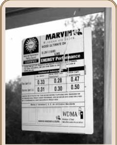
Energy label reports tested values for heat loss (U value), blocking solar heat gain (SHGC) and transmitting visible light (VT)
