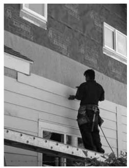
Fiber-cement composite siding is durable and low-maintenance
