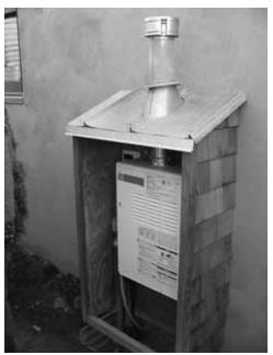
A tankless water heater eliminates stand-by heat loss of conventional tank-type heater
