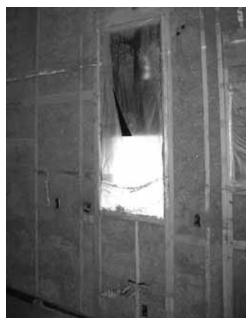
Spray-in cellulose insulates and stops air leaks
