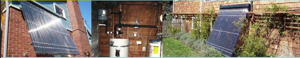
Collectors can be mounted vertically or horizontally, although the goal is to maximize the unit's exposure to the sun.
