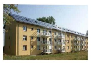
This method only works with evacuated tube collectors, which are generally more efficient at high operating temperatures than flat plate collectors and - probably even more importantly - are resistant to freezing in winter time due to the vacuum insulation around the collector pipes. The exterior piping of the collector loop should be kept as short as possible, as freezing in the pipes and collector is prevented by occasionally circulating a small amount of heat from the store.
