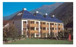
This means that pipe connections from the collector into the apartment are very short. A simple controller could allow the electrical heating element to heat the store only after sunset, if there was not enough solar radiation to bring the store to the desired temperature.
