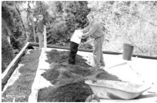
Patrick Carey and Katie Spataro spread soil on the Sproull-Radke workshop roof after the waterproof membrane and root barrier have been installed.
