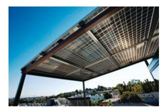
Photovoltaics integrated into awnings and attached to trellises collect solar energy while helping provide shade.
