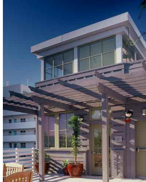
Interior (left) and exterior (right) of the very green Natural Resources Defense Council offices in Santa Monica, Calif.
