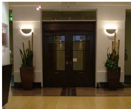
Reused doors and relights, bamboo flooring, low-VOC paints and adhesives, FSC-certified wood, formaldehyde-free MDF reception desk with non-toxic finish and energy-efficient lighting were a few of the green features incorporated into Otak's Seattle office renovation.
