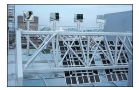
**Roof mounted mirrors, heliostats, direct light into the building through a skylight.** Photo Courtesy of Genzyme Corporation
