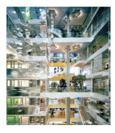
Andover Continuum floor controllers interface with lighting components to yield significant savings by eliminating the need for a separate network system to handle the lighting. In addition, TAC's Smart Sensors give employees individual room control for HVAC and lighting.
