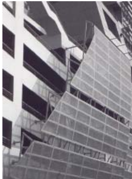
Sunscreens/Shading device fit like 'loose-clothing' on the structure of the tower.
