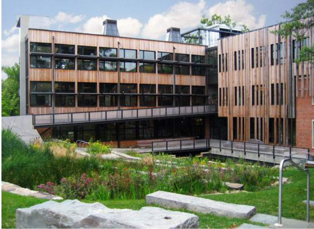
(View from top of the wetland terrace towards the new building extension. Photo by Andropogon Associates.)
