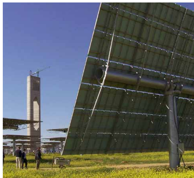
121 m 2 heliostat at Abengoa PS10 power tower, Spain 11
