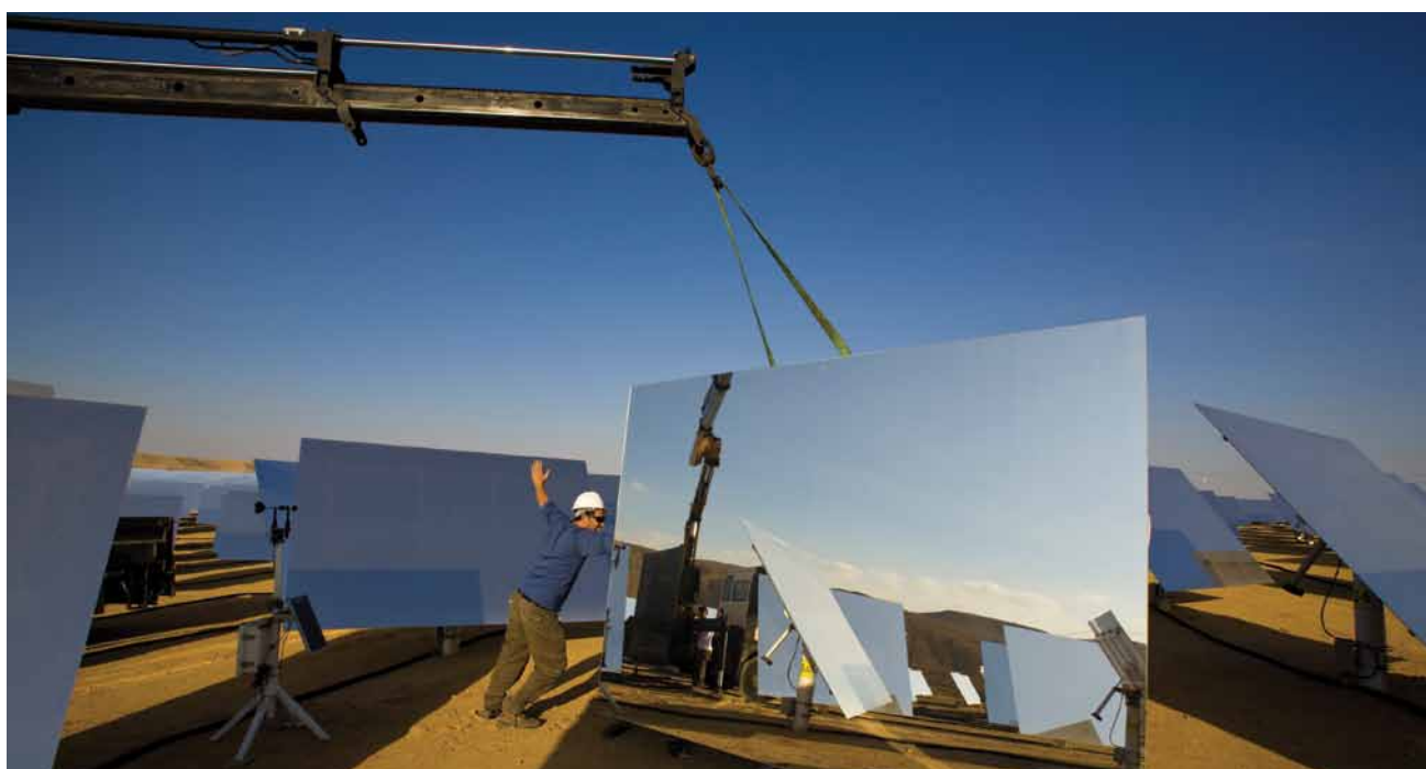
Construction workers installing heliostats at a Brightsource solar thermal power tower 42
