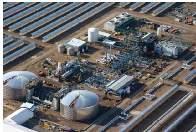
Molten salt storage tanks, Andasol 1, Spain
