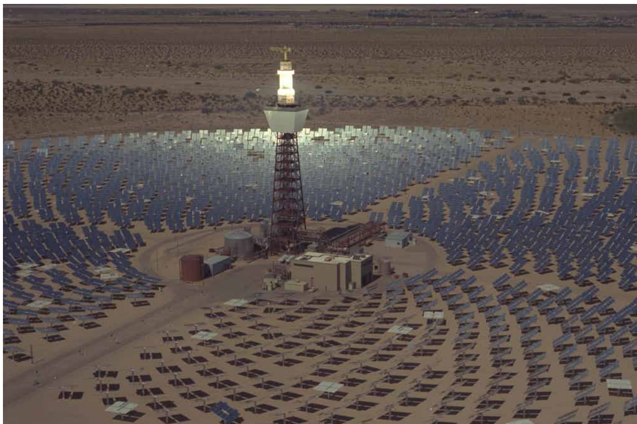
Solar Two in operation at Daggett, California, 1999 2 . Molten salt tanks are the silver pair at base of tower.
