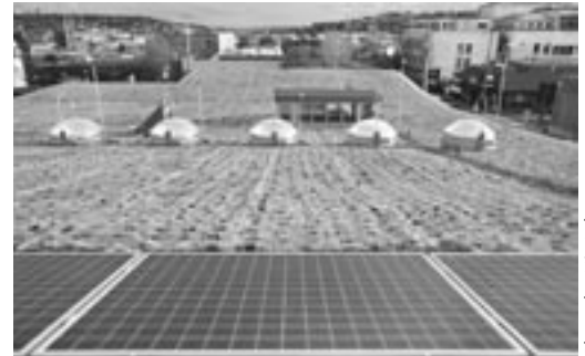
Green roof and solar panels.
