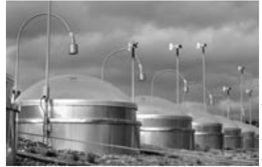
Skylights and anemometers.
