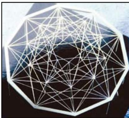
Figure 12: HB Cable Dome System.
