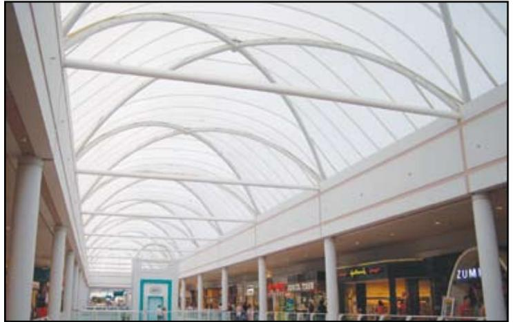
*Figure 10: Silicone Coated Fiberglass Roof at the Poughkeepsie Mall.*
