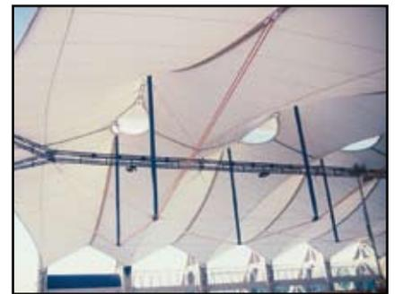
*Figure 11: Flying Struts at San Diego Convention Center.*
