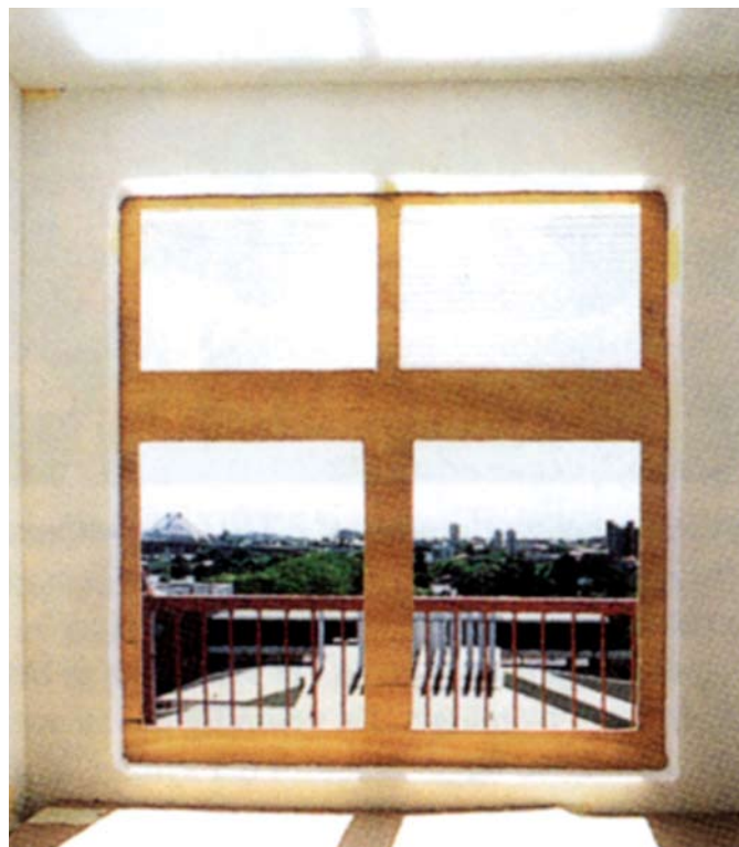
Holographic window reflecting sunlight to the roof in order to enhance the use of daylight.
