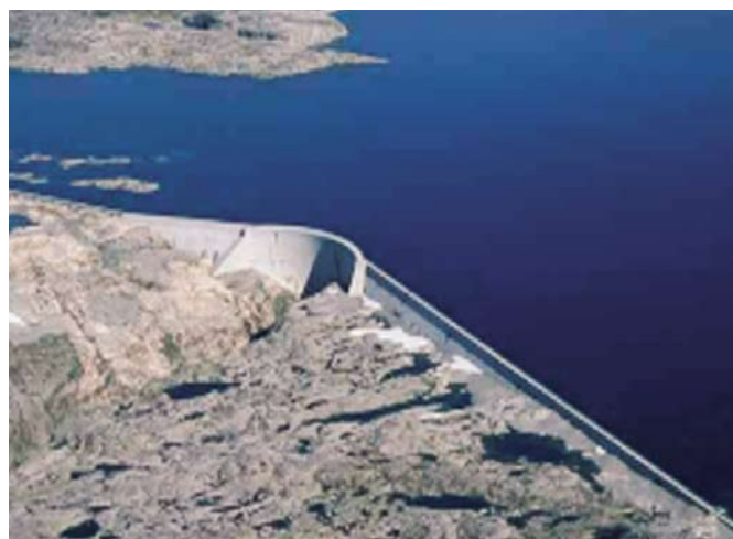
In Norway there has been built more than 330 large dams (higher than 15 metres). Here the Forresvass dam which is a combined gravity and arch dam. Photo: Statkraft.
