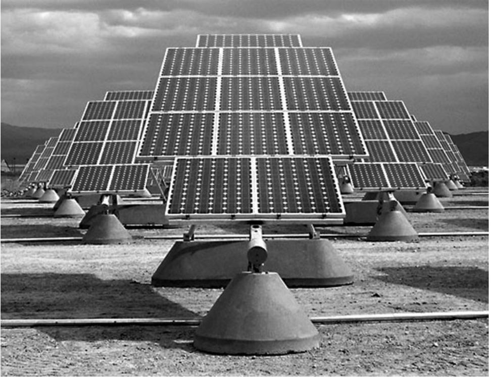
**Figure 3.55** SunPower T20 single-axis solar power-tracking system. *Photo courtesy of SunPower.*
