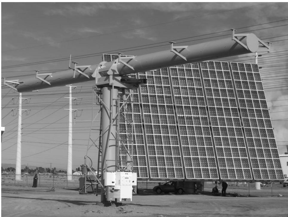
**Figure 3.22** Amonix MegaConcentrator hydraulic arm assembly. *Photo courtesy of Amonix.*
