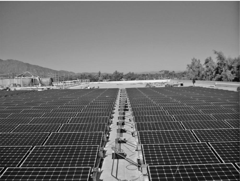
**Figure B.17** Nonpenetrating-type roof-mount-solar power assembly. *Photo courtesy of DWP Solar.*
