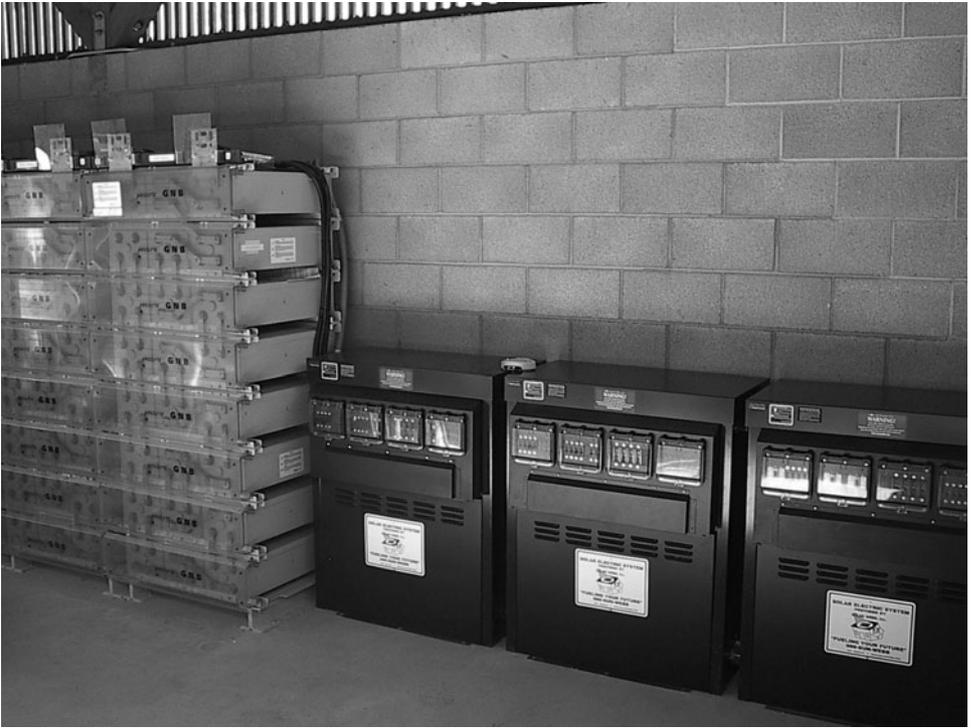
**Figure 3.43** Deep-cycle battery packs. *Photo courtesy of Solar Integrated Technologies.*
