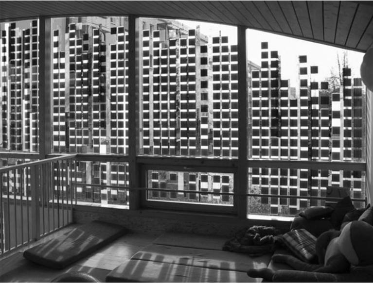
**Figure B.10** Building-integrated solar power used as decorative curtain wall. *Photo courtesy of Atlantis Energy.*
