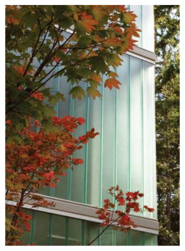
After some research, it was determined that Pilkington Profilit translucent linear channel glass system was a natural fit for the project. The product takes advantage of borrowed daylight, thus reducing the need for artificial lighting. It is available in a variety of colors and textures with varying translucency, and works well with the environment and surroundings. In addition, it is one of the only systems to allow floor to ceiling glass with no intermediate spans.
