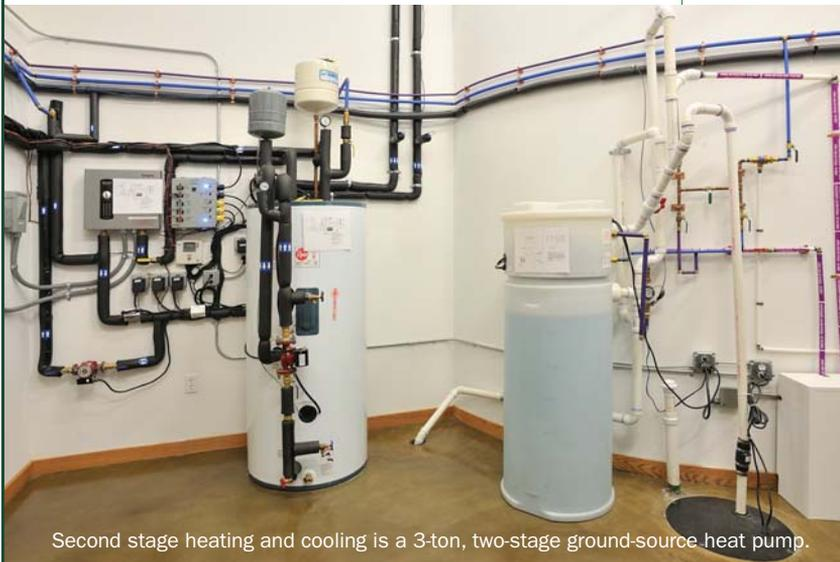
Second stage heating and cooling is a 3-ton, two-stage ground-source heat pump.
